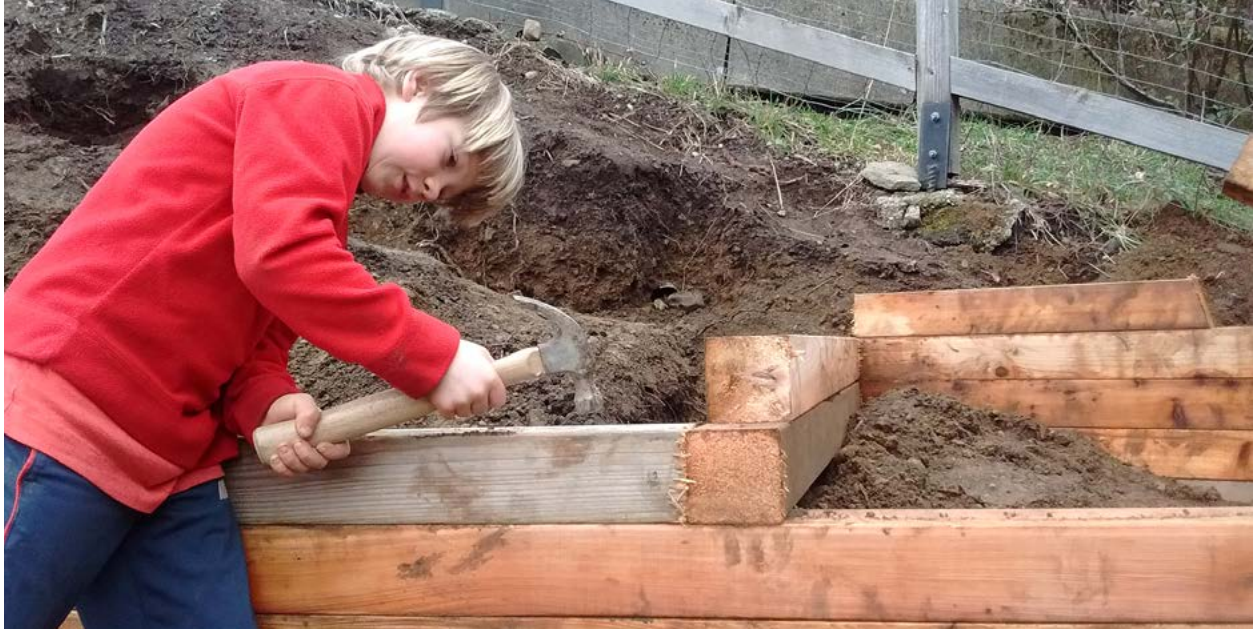
building garden terraces at SSE
